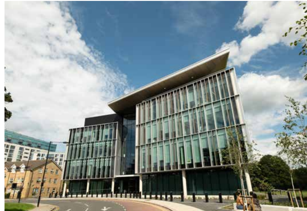
Metaswitch offices, Enfield Town
